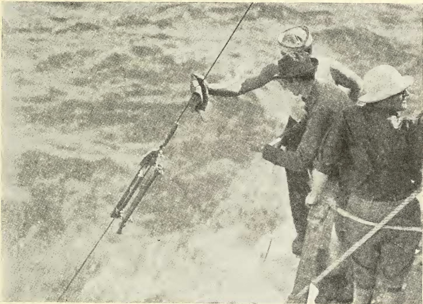
Fig. 26. Water bottle coming to the surface showing messenger resting on the wire above the machine.
